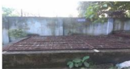
Rain water harvesting @ supplier site Jamshedpur
