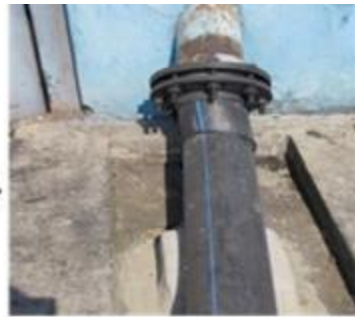
WATER PIPE FROM SHED TOP
