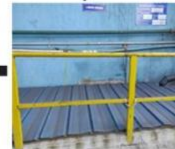
MAIN PIPE LINES TO CHAMBER
