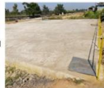
PRIMARY STORAGE TANK
