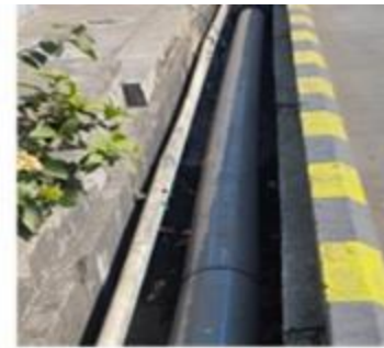
MAIN PIPE LINES TO CHAMBER
