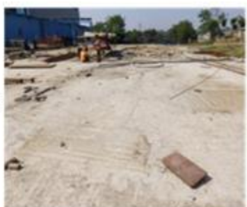
SECONDARY STORAGE TANK
